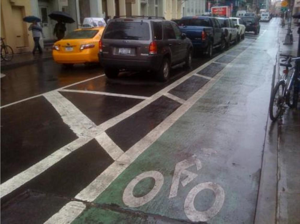
Note the space between the bike path and the passenger side of the parked cars in order to prevent cyclists being "doored" by people exiting cars on the passenger side (and to prevent passengers being "biked").
